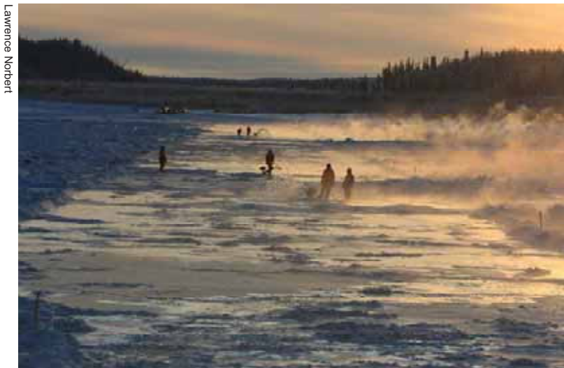
Workers flooding river ice to build it up and smooth it out for an ice crossing on the Dempster Highway
